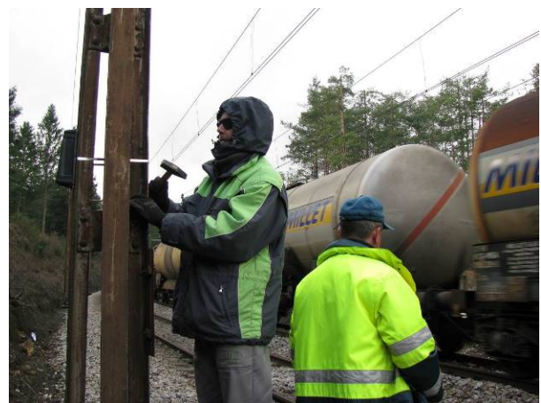
Figure: Installation of acoustic deterrents on two types of electric poles along railway sections (photo: M. Zaluberšek).
