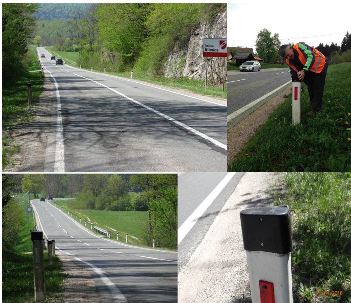
Figure: Acoustic deterrents installed along the main road Ljubljana – Kočevje (photo: M. Zaluberšek).
