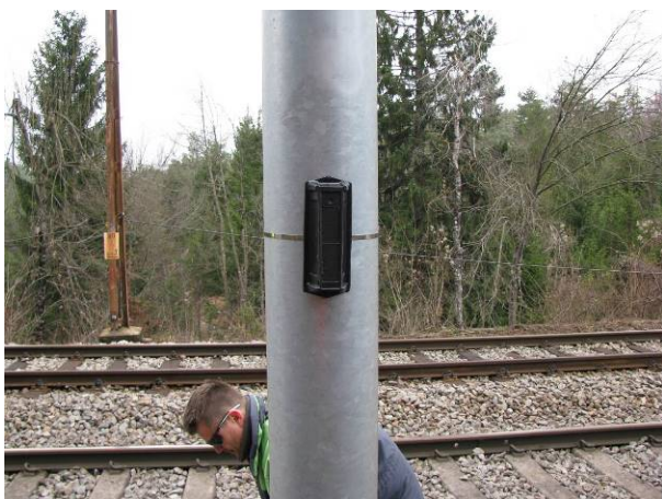
Figure: Installation of acoustic deterrents on two types of electric poles along railway sections (photo: M. Zaluberšek).
