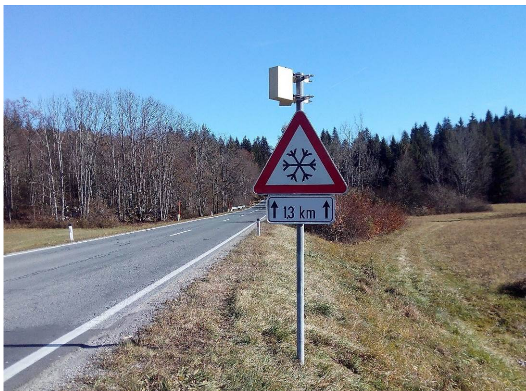
Figure: Traffic counter placed on the pole of traffic sign near Dolenja vas (Jasnica).
