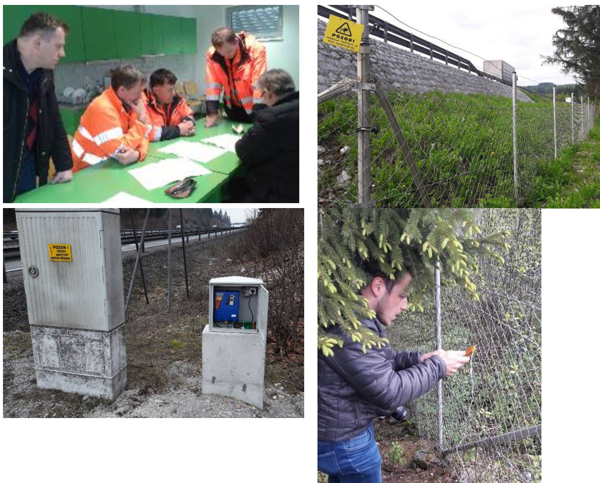
Figure: Electric fence installed along the Ljubljana – Koper (A1) highway (photo: S.Petkovšek, Z.Pavšek).
