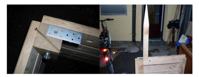
3. Install the composter lid with the hexagonal-head screws. Use a ratchet and a 17 mm socket wrench.
