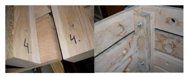
Use clamp bolts, washers and wing nuts to join the corners. The screw holes are already made.
