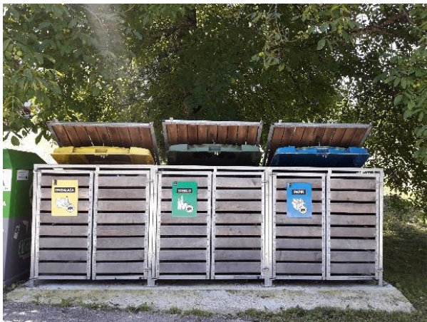
Figure 7: Covers of the garbage containers are properly attached to the cover of the housing – they open simultaneously.
