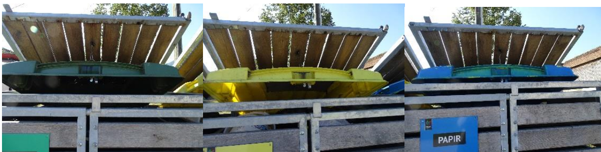
Figure 23: covers of the garbage containers are properly attached to the cover of the housing – they open simultaneously.
