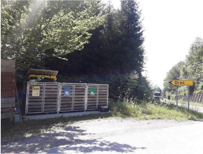
Figure 20: “Bear-proof” garbage housings for large (~ 1000 litre) containers are located right next to the regional road Kočevje-Petrina.
