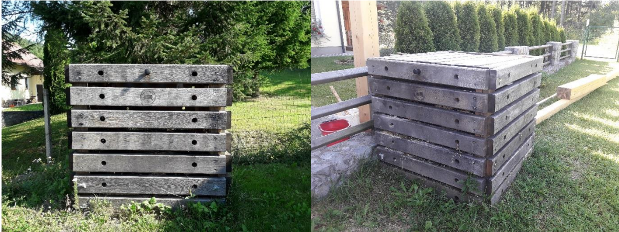
Figure 9 and 10: Good operation and condition of the compost bins on the location.
