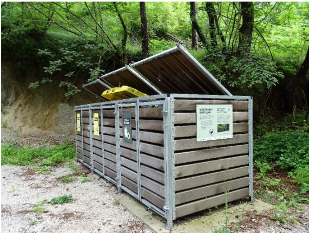
Figure 3: Missing cover pins of the two newly replaced garbage containers' cover.
