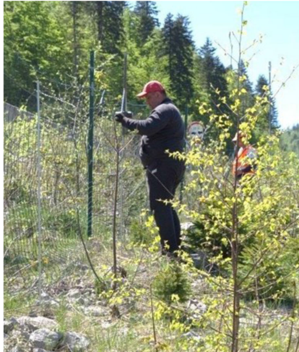
Figure 2: Preparing the location for the implementation of the electric fence.
