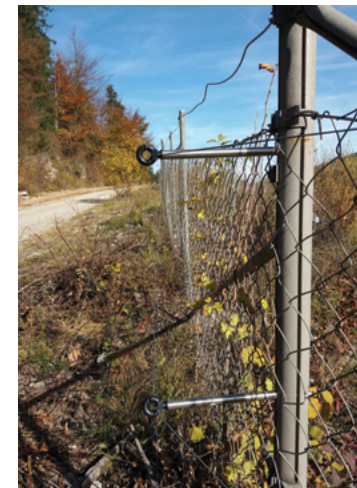
Electric fence installed on Primorska highway between Logatec and Lom to reduce bear and other wildlife collisions with vehicles.
