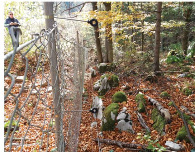
Electric fence installed on Primorska highway between Logatec and Lom to reduce bear and other wildlife collisions with vehicles.
